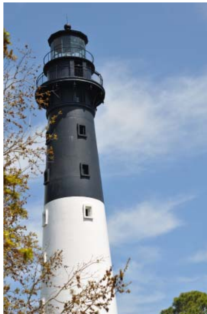
Hunting Island Lighthouse photo by Jay Leach
